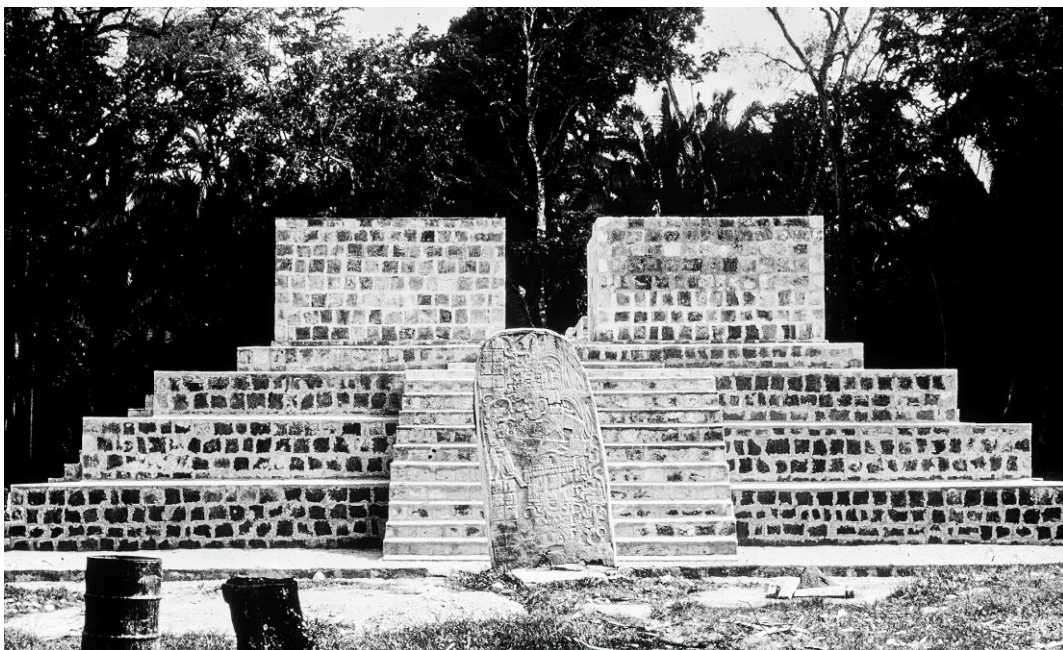
Figure 6.9. Ceibal Structure A-3: top, before excavation; bottom, after reconstruction in 1964.
