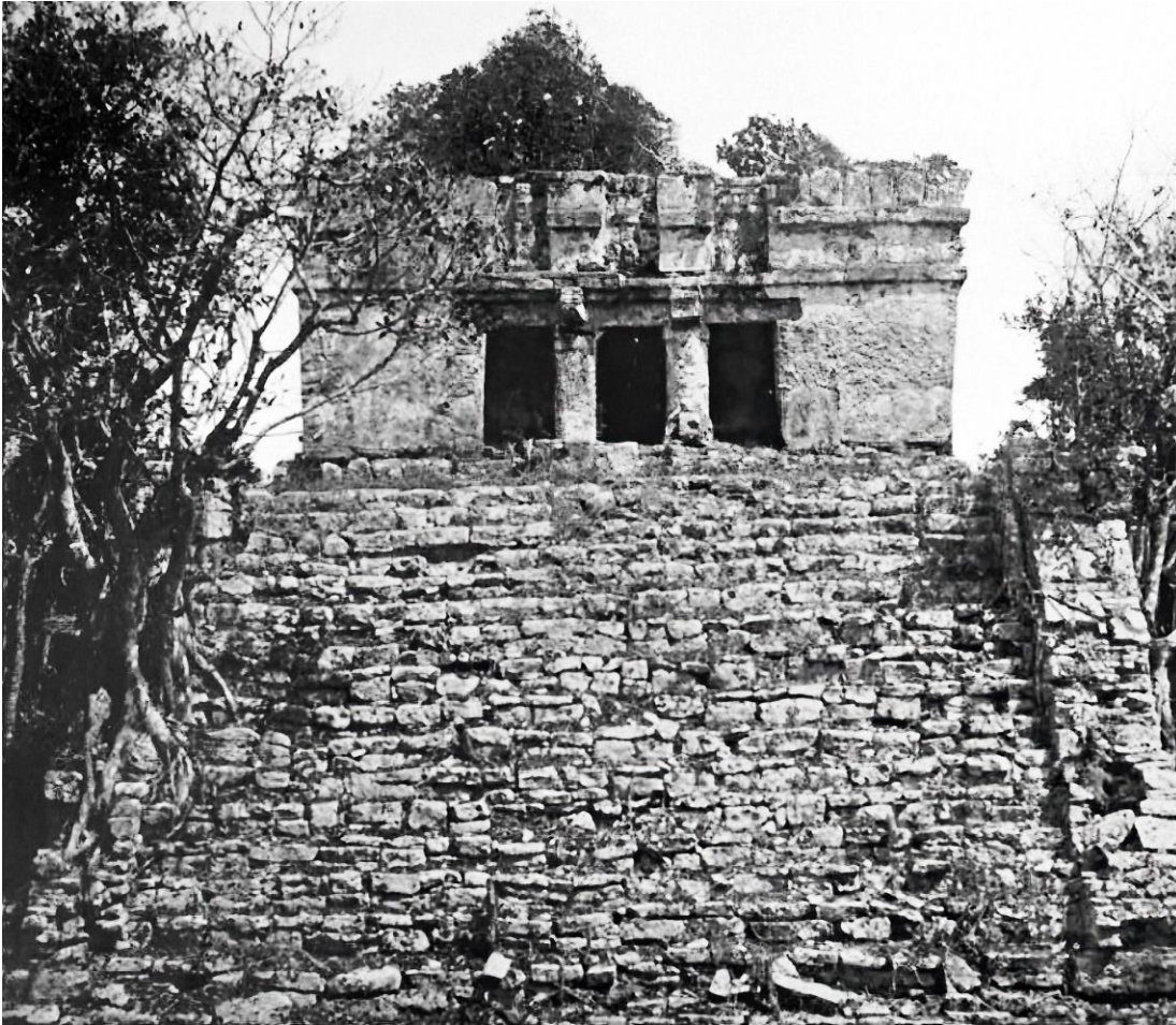
Figure 19.7. The Castillo in 1916. The chief agent responsible for the destruction of the ancient Maya cities is not the hand of man, disastrous as that has been, but the mighty strength of an irresistible vegetation. Large trees, striking their powerful roots deep into the foundations of temple or palace, literally rend it stone from stone, the masonry collapses, and denigration follows. This photograph shows the destruction wrought in the past seventy-five years. The cornice of the main temple, the balustrades, and stairway appear to have lost a few stones, but otherwise the Castillo looks much as it did in Stephens' time.
