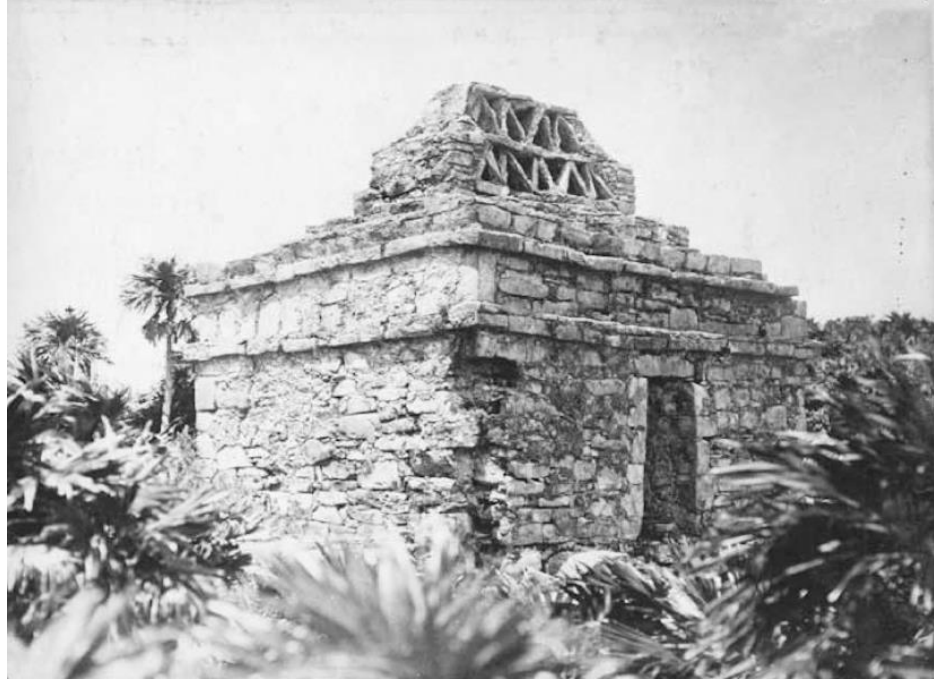
Figure 19.13. The small temple, standing a few hundred yards outside the Tulum walls to the north, presents a feature common in Maya architecture—namely, the roof comb, a wall purely decorative in purpose and usually embellished with an elaborate design in stucco.
