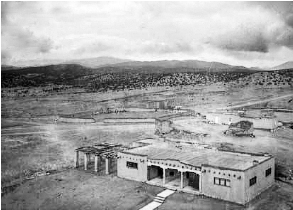
Figure 1.2. Morley's house shortly after his 1909–10 renovation.
