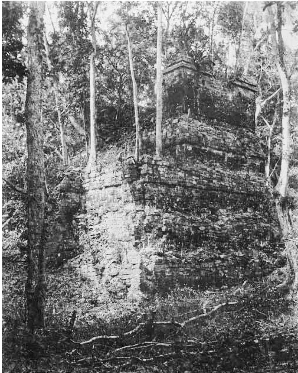
Figure 8.1. Southwest corner of Postclassic Structure C at Topoxte, which since has been reconstructed.
