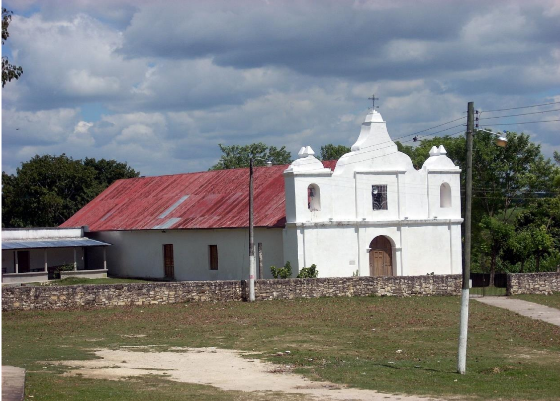
Figure 7.13. Refurbished Colonial church in Dolores built in 1708.
