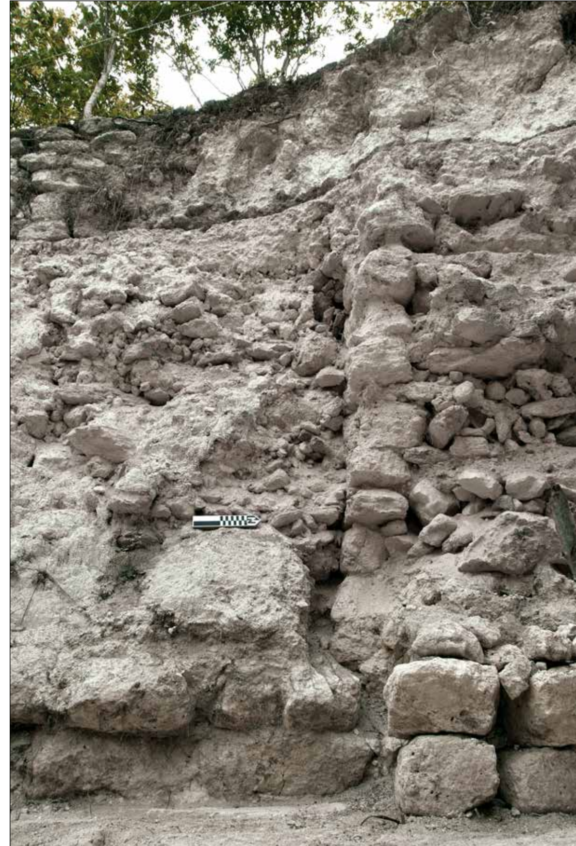
Figure 2.47. Fill above the Temple of the Night Sun, with retaining walls to prevent lateral displacement of the newly added bulk for Str. F8-1-2 nd . Photo: Arturo Godoy.
