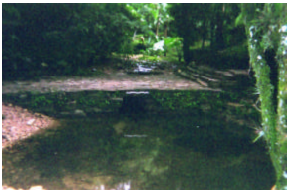
Figure F 4 – Palenque's only fully functional bridge, OT-B1.
