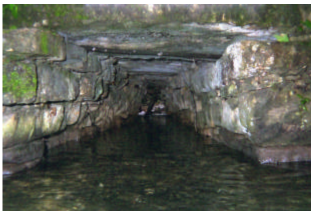
Figure F 5 – The vaulted channel that allows for water passage beneath the bridge.
