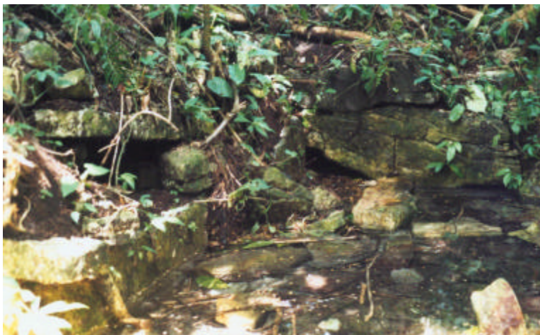
Figure C 6 – A view of PB-P1. The overflow drain is on the left edge of the photo.
